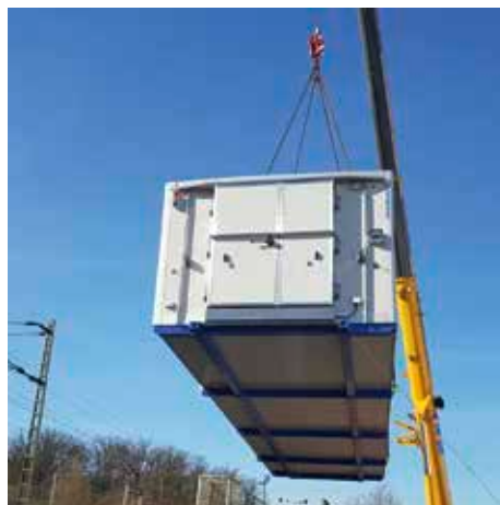
Frei Haus: Transportables Kühllager am Haken. / Transportable cold storage on a hook.
